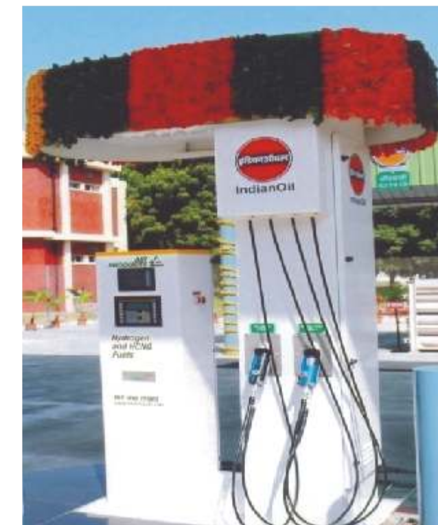
India's 1st HCNG Dispensing Station
